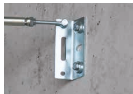
Fixing of brackets and console bearers
